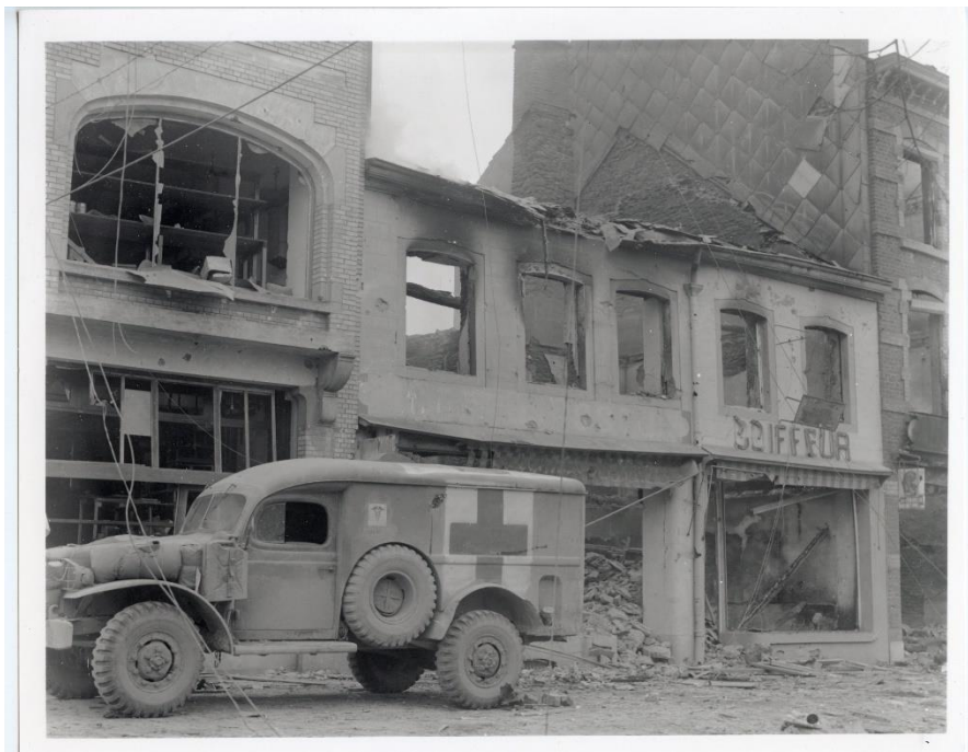
War-time damage in Bastonge.
