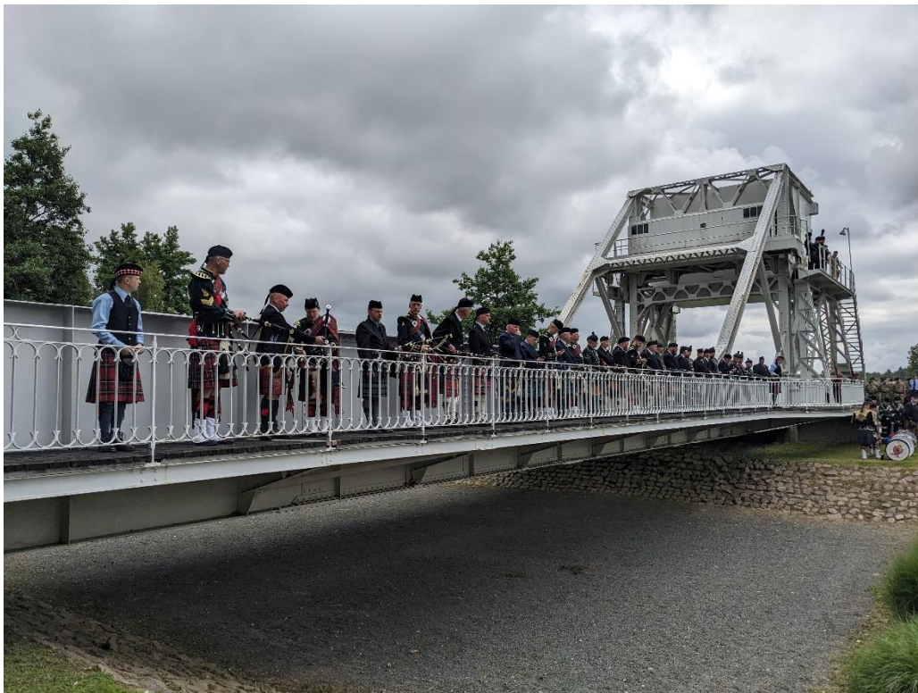
Members of a pipe band on the original Pegasus Bridge during the 2024 80 th Anniversary Commemorations
